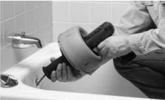
**Figure 6 – Push Cable Down Drain Line**
